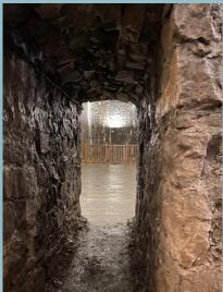
vaulted chambers built by Brunel and his team almost 180 years ago. Stalactites drip from the ceilings and in the first vault you can clearly see how the abutment is built around the bedrock of the cliff face.
